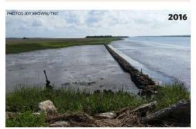
The reef was installed in April 2016 and made of wooden pallets, Oyster Castles™, and bagged oyster shell. Prior to its installation, heavy wave and boat activity had caused the marsh to erode into a U-shape.
